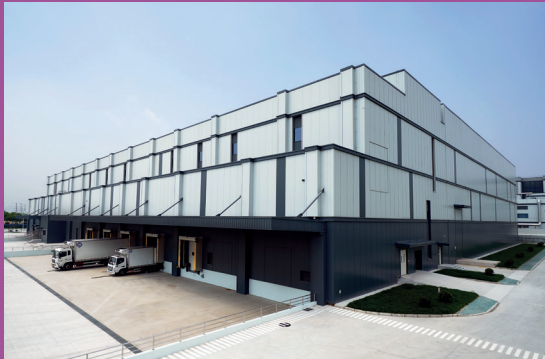
Merck, China OSD Manufacturing, Packaging and Logistics Facility
